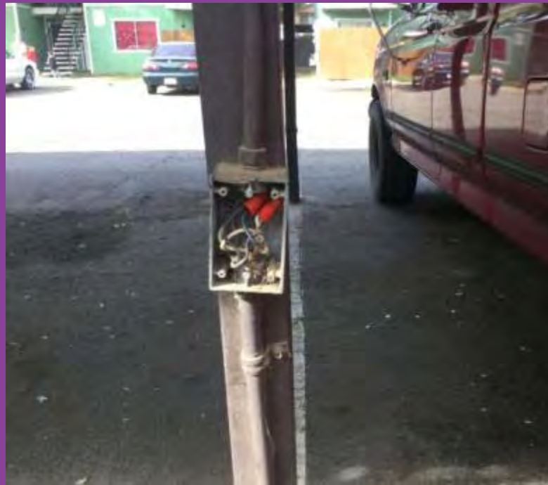
Exposed Wiring
